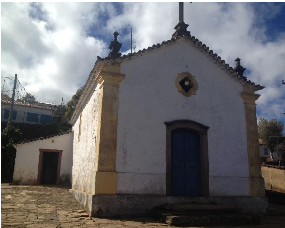
Figura 26 Fachada Principal Fonte Thatiane Rocha 2017
